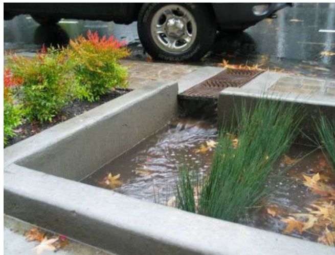
A photo of a rain swale, an important stormwater management method which naturally filters some contaminants from runoff.
